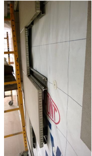
Figure 4: Limestone Panel System | Quaid Spearing
