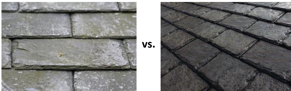
Figure 2: Slate Shingles vs. Rubber Shingles | images courtesy of Google images
